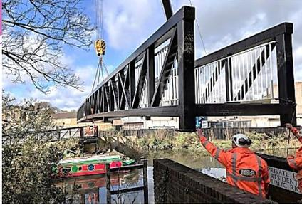
Works to replace the footbridge across the canal have made significant progress in the last week, with the main sections being lifted into position by an impressively large crane.
